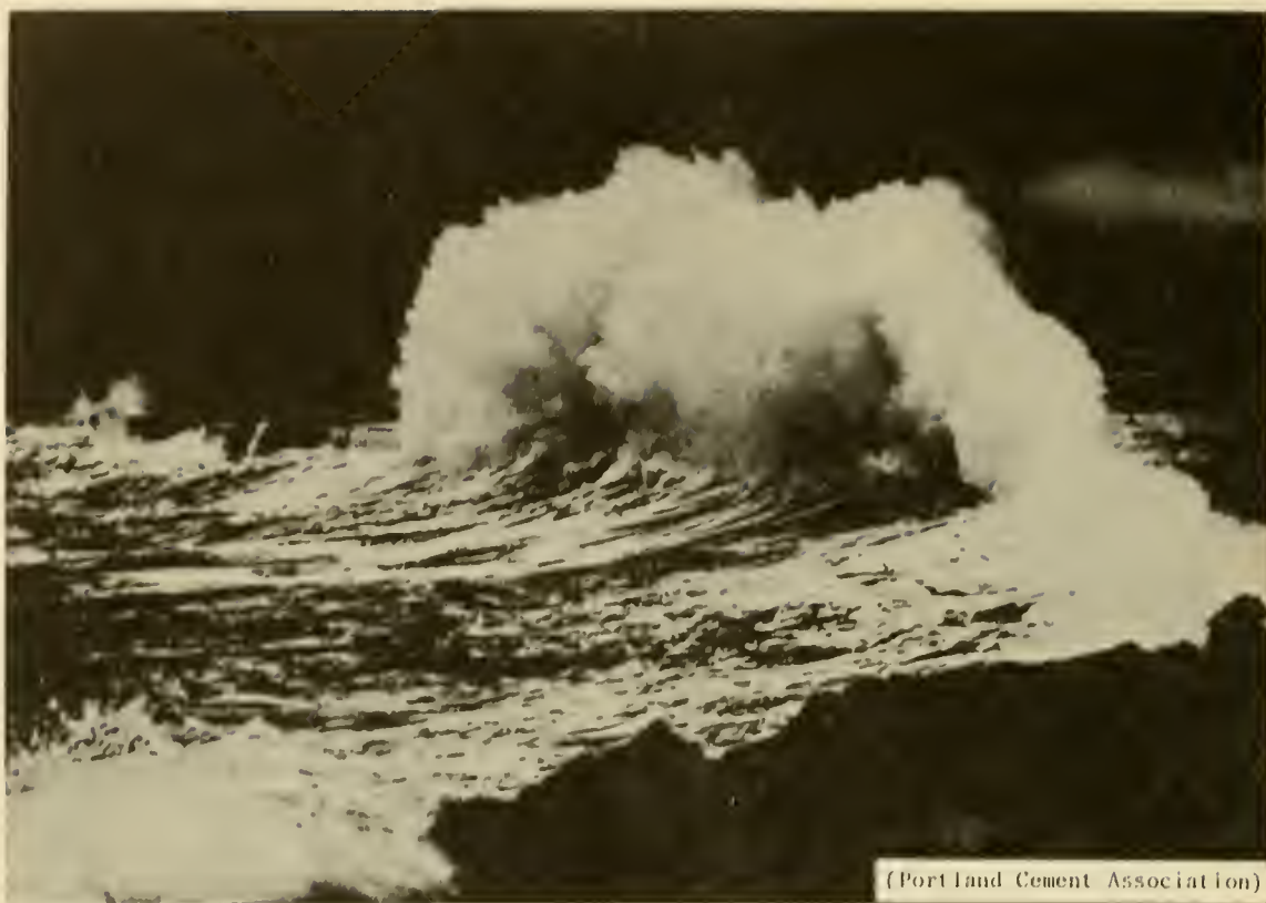
Figure 1-5. Large Waves Breaking over a Breakwater
