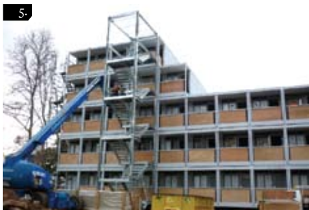
1-5. The pre-fitted containers assembled on site. 6-8. Finished exterior and interiors. Photos: courtesy QuickSmart Homes.
