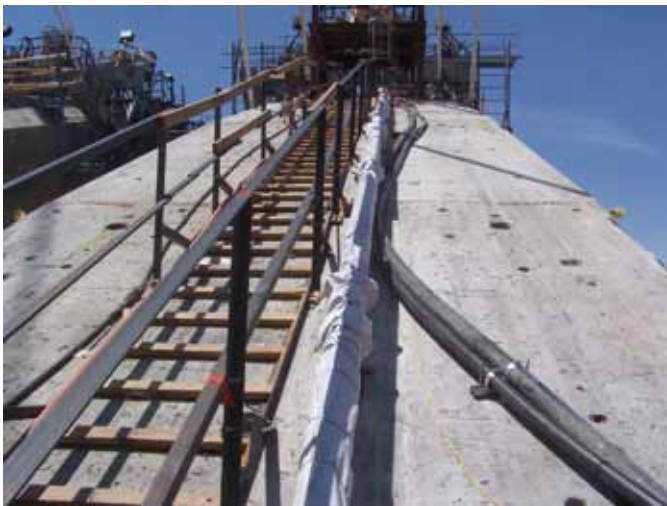
Fig. 3: The concrete slickline wrapped in burlene. Soaker hoses inside the burlene delivered chilled water to the exterior of the slickline in an effort to reduce concrete heat gain during pumping (photo courtesy of Obayashi/PSM JV)
