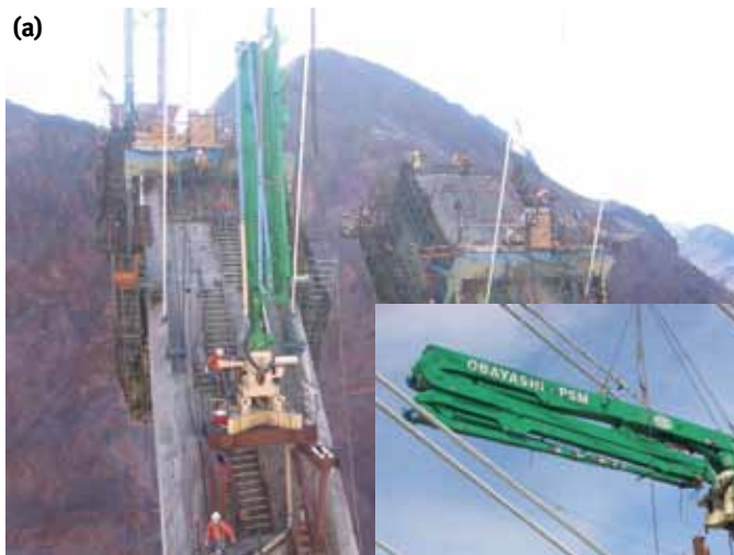
Fig. 7: (a) The placing boom and platform on the Nevada-side arch cantilevers; and (b) placing boom being relocated (photos courtesy of Obayashi/PSM JV)
