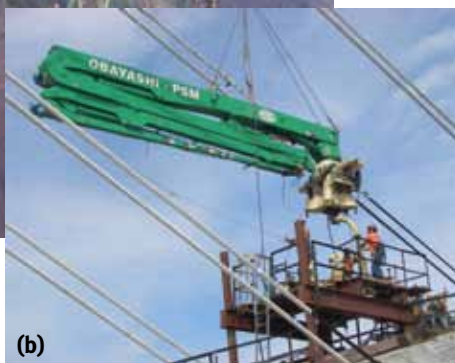
Fig. 7: (a) The placing boom and platform on the Nevada-side arch cantilevers; and (b) placing boom being relocated (photos courtesy of Obayashi/PSM JV)
