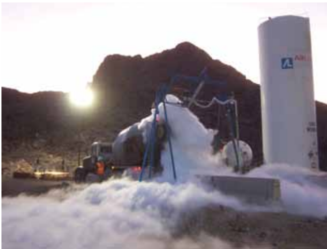
Fig. 2: Liquid nitrogen being injected into a concrete truck (photo courtesy of Obayashi/PSM JV)
