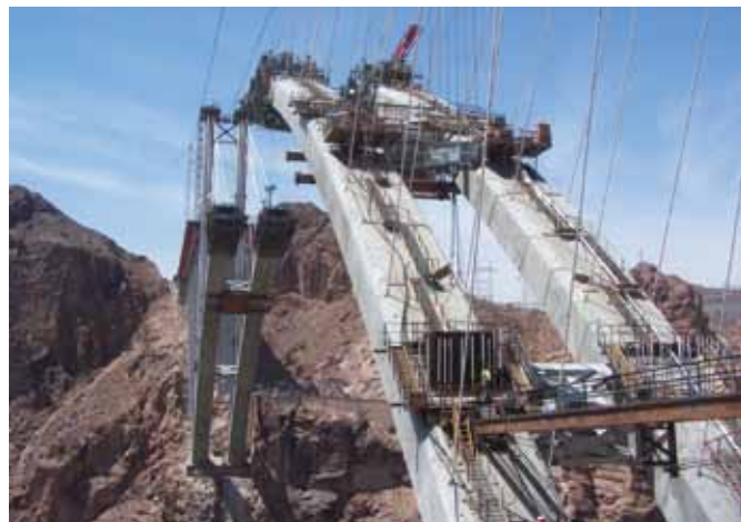
Fig. 6: A view up the Arizona-side cantilevers. The concrete slickline can be seen just off-center of the cantilever on the right (photo courtesy of Obayashi/PSM JV)
