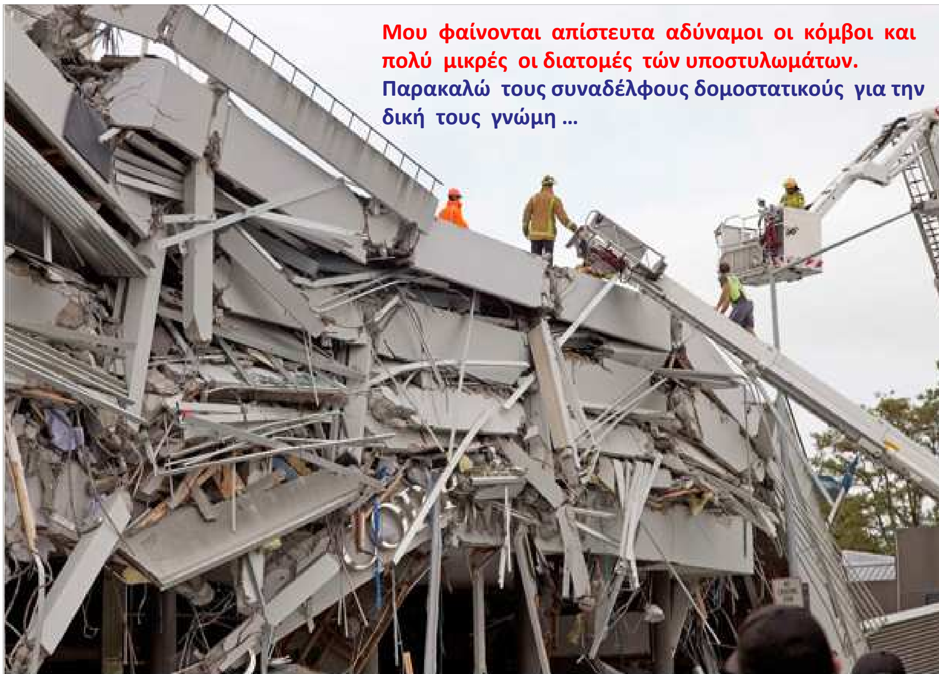
The Pyne Gould Corporation building in central Christchurch after the 6.3 earthquake, February 22, 2011. Photo / Simon Baker
