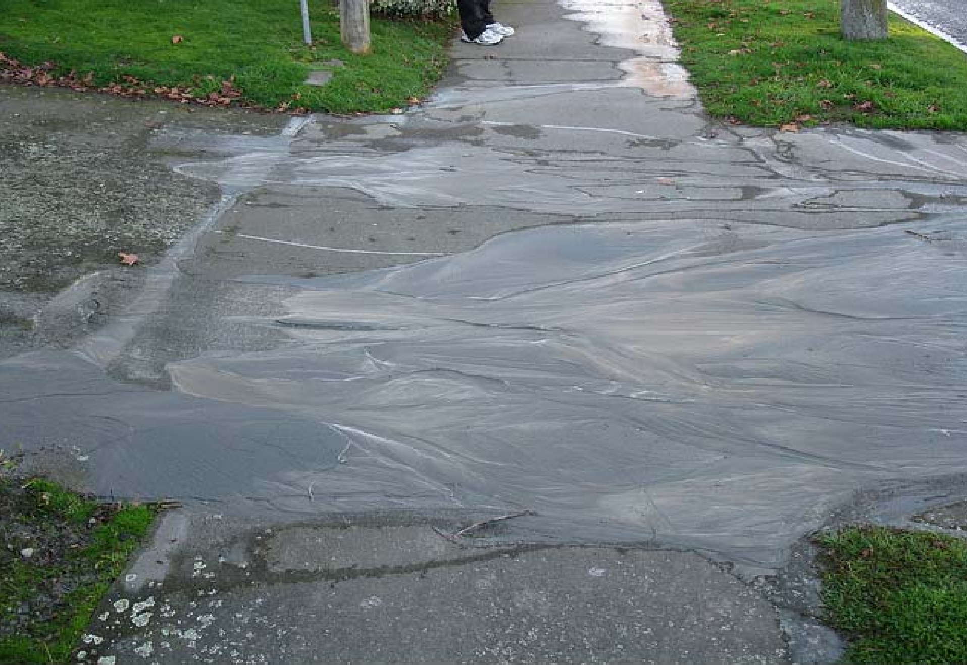
Sand coming through the ground
