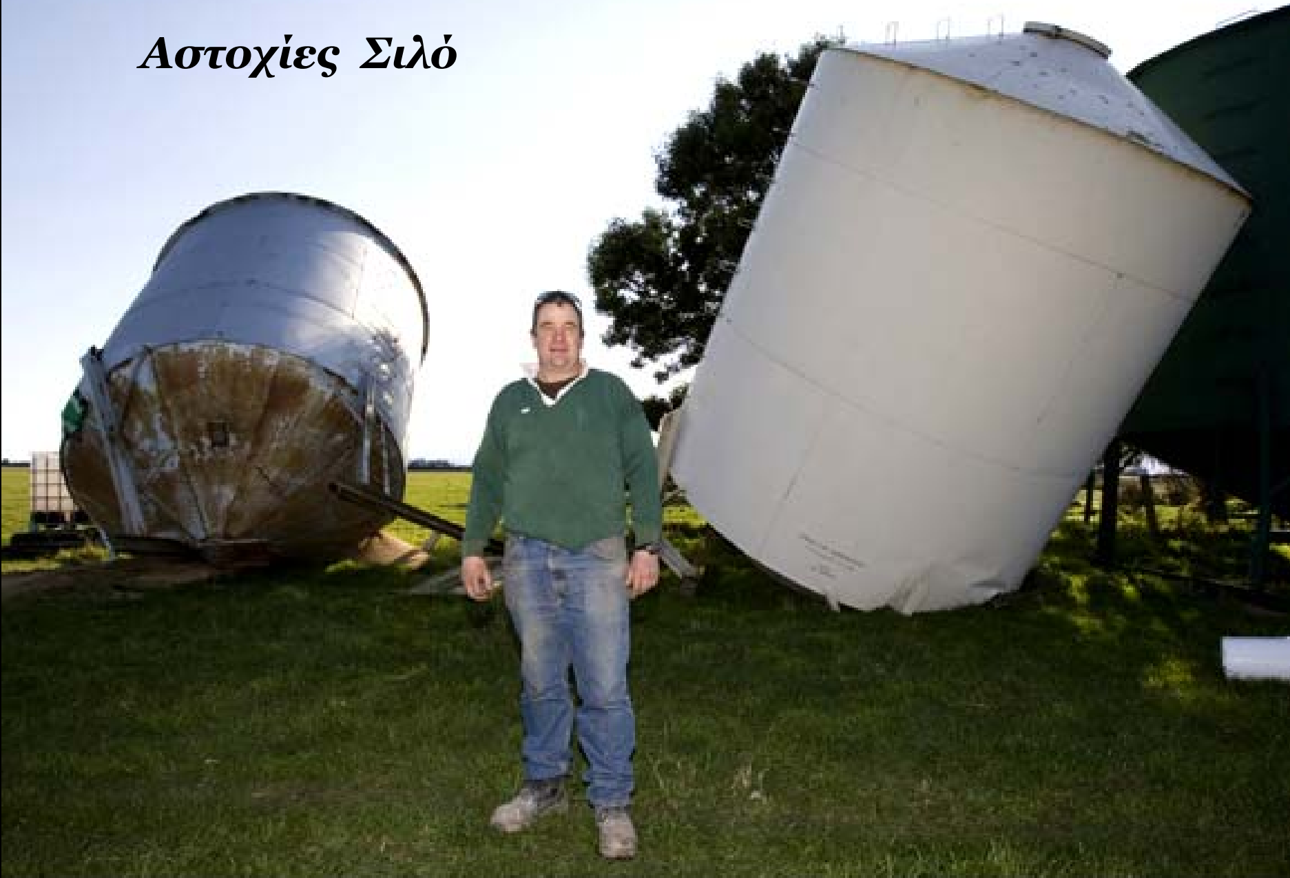
George Redmond with the 35 ton wheat silos that collapsed on his property at Courtenay, east of Darfield. Photo / Mark Mitchell
